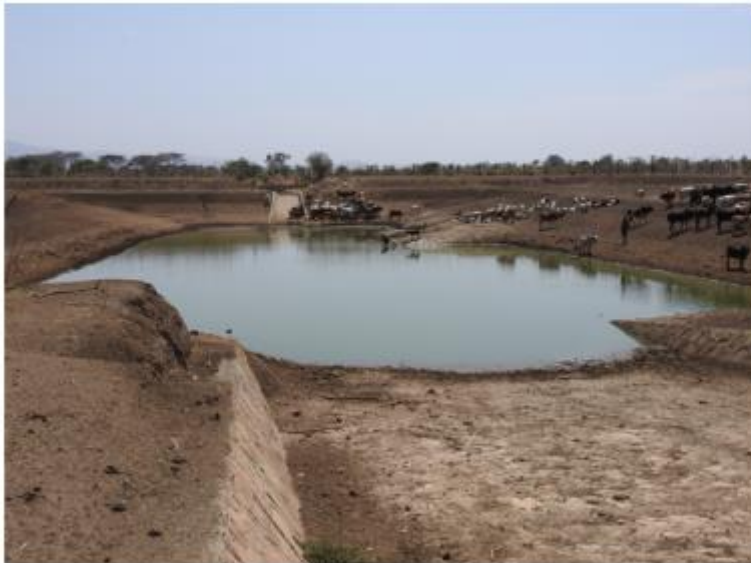
B) Valley Tank (3 photos) – cattle entering at wrong points while water committee member was present.
