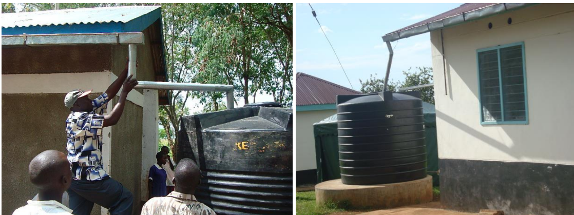
Plate 5: Roof Rainwater Collection System in Sauri MVP
